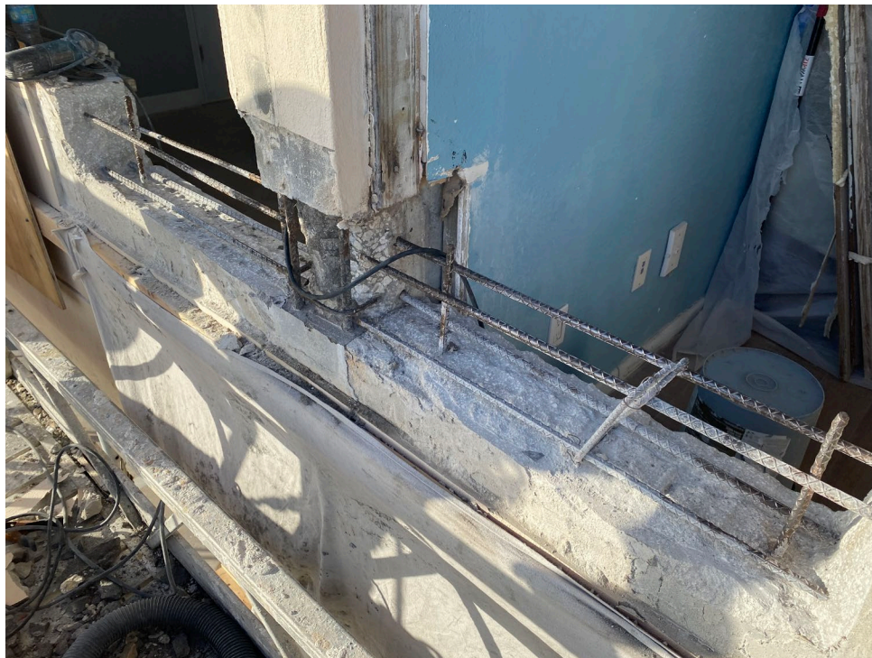
Picture 4: Unit 108 and 109 window sill repairs
