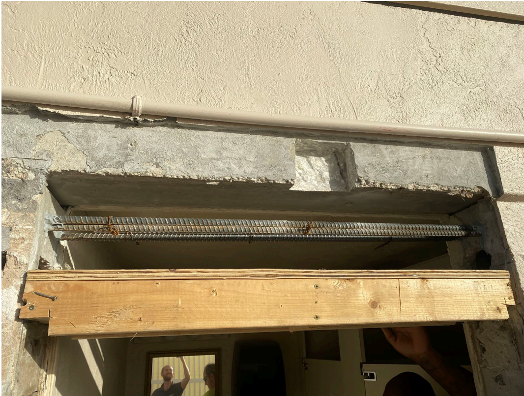
Picture 3: Header repair at Women's bathroom
